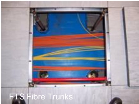
Under Floor Cable Containment
